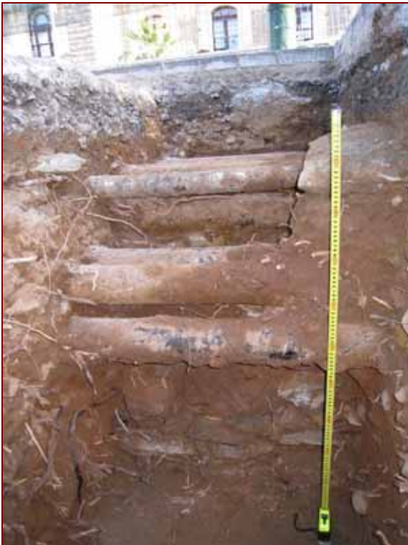
Figure 5: A view facing south of the wall in Trench E. Note the proximity of the service pipes to the wall. 1m scale
